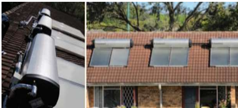
Figure 7: Residential thermosiphon SWHs in Western Cape, South Africa
